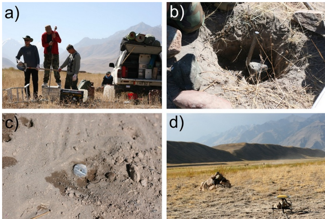
Figure 5: Installation of marker WA04 in alluvial sediments, that consists of a) a steel rod that is hammered and b) cemented into the ground. c) A small hole defines the marker for the d) GNSS instrument set up that is stabilized with smaller rocks.
