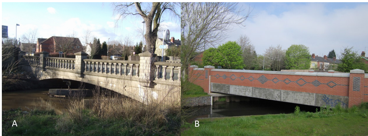
Figure 5: (A) The previous Dogpool Lane Bridge across the River Rea in which reinforcement blocks under bridge constricted high flows. (B) Replacement bridge in 2012 (reinforced without blocks) to allow high flows to continue downstream. Photos published with permission from the Selly Park South Neighbourhood Association (SPSNF, N.D.)
